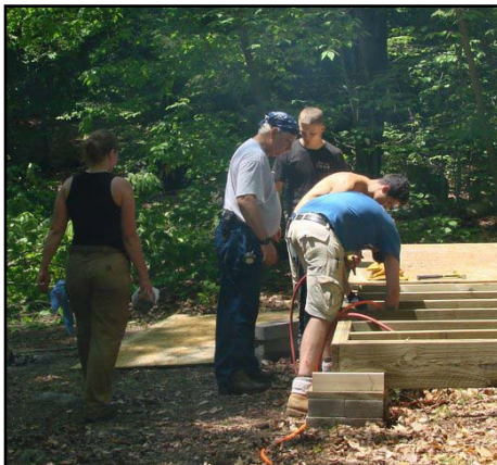
New Lean-to Construction at Camp Buckskin
