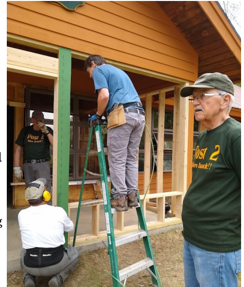
Tim Haag, Bill Daley and Bill Brucker Working on the Newton Hall Front Porch
